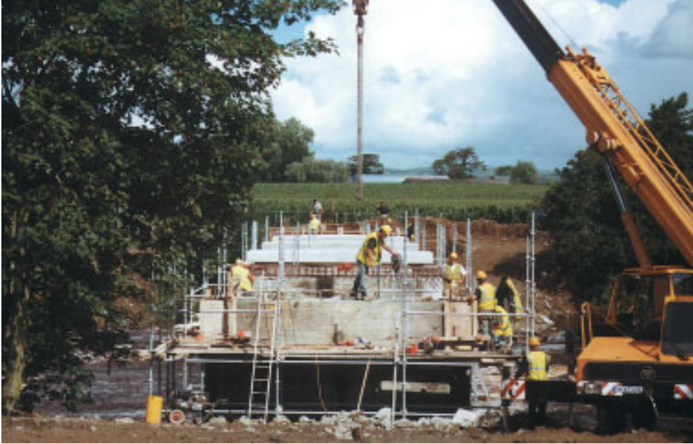
New bridge construction on the River Feale in Co. Kerry
